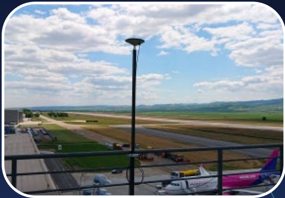
GNSS Monitoring and Interference Detection in Romanian Airports (RO)
